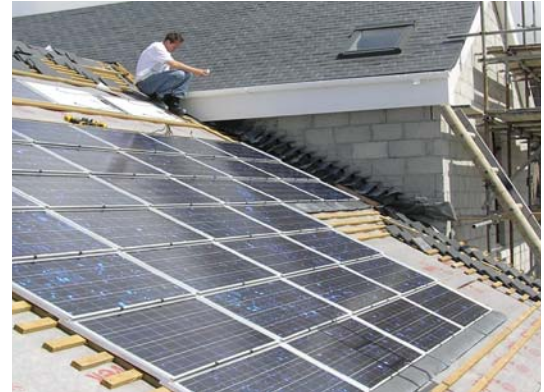
Fitting of solar PV on the roof of the centre
