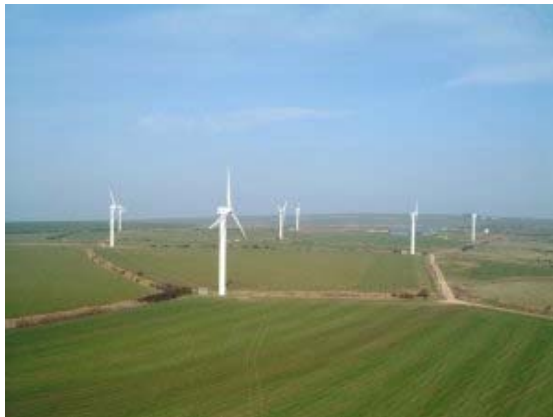
Delabole wind farm
